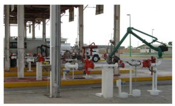
Unloading arms can be assembled and manufactured in accordance with client needs, or can arrive integrated in skid type equipment.
